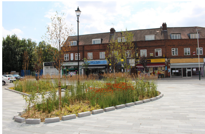
Example of rain garden to provide sustainable drainage and create a visually attractive barrier between vehicle and pedestrian areas
