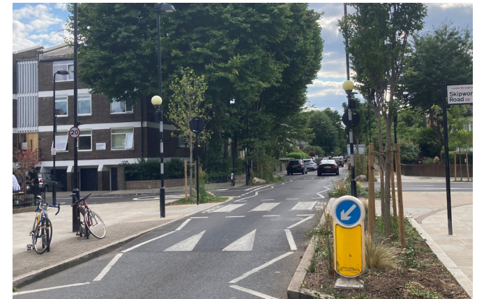
Example of raised zebra crossing with planting and cycle stands which prioritises pedestrians and encourages vehicles to slow down
