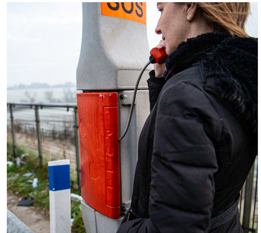
Emergency roadside telephone.
