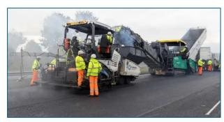
The trial was delivered in collaboration with Tarmac, Kier, HW Martin and other suppliers. We achieved a 75% reduction in carbon emissions compared to traditional resurfacing. This is a saving over 260 tonnes of carbon. Innovative techniques used to make this possible. We use warm mix asphalt,
