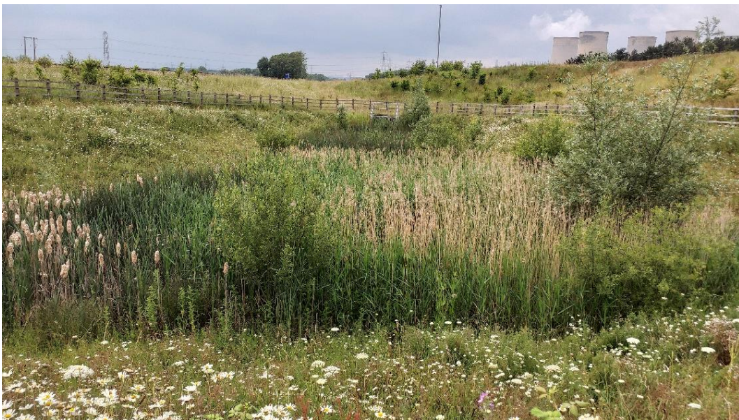
Figure 11 Overgrown balancing pond at West Leake junction
