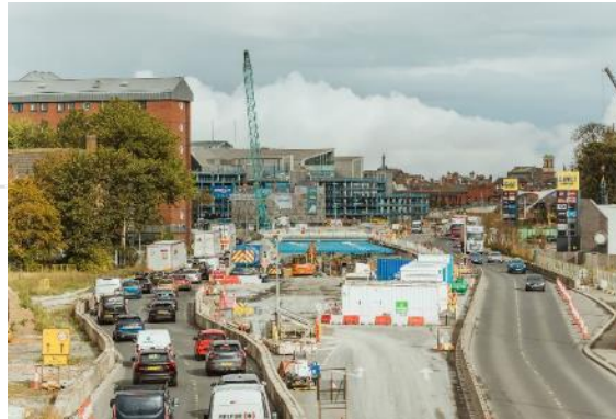
Figure 22: Example of Temporary Traffic Management on the SRN
