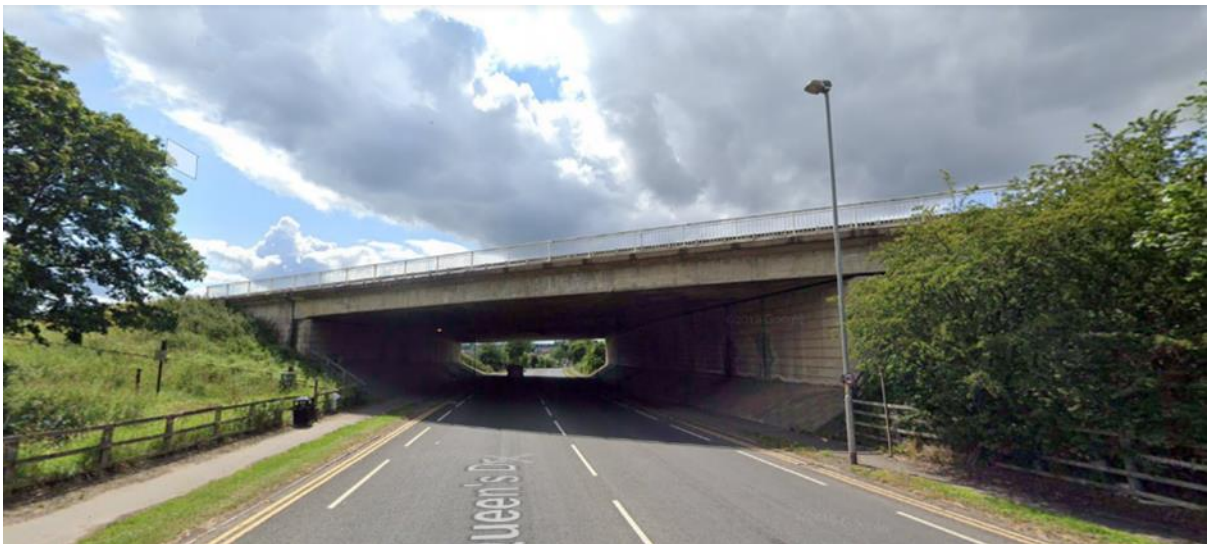
Figure 5.13 Queens Drive Bridge viewed from the east (source: Google Streetview, August 2020)
