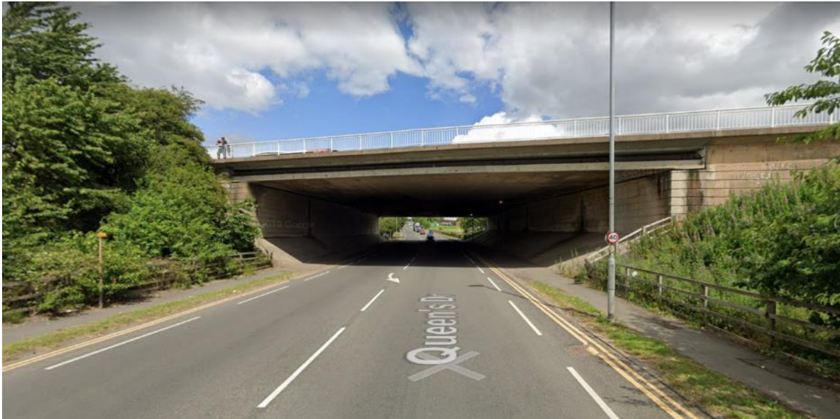
Figure 5.12 Queens Drive Bridge viewed from the west (source: Google Streetview, August 2020)
