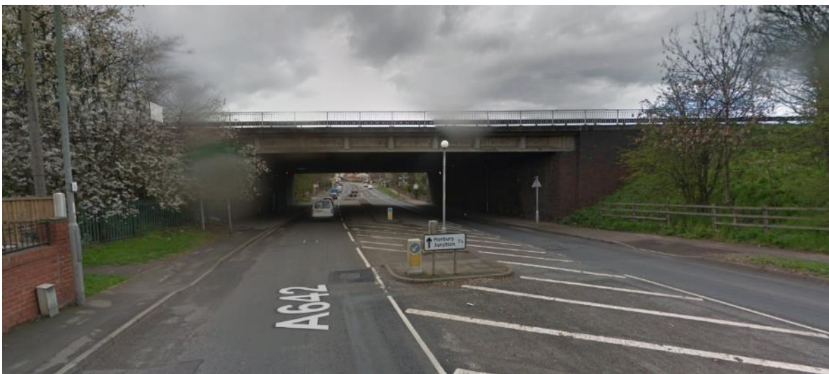
Figure 5.9 Horbury Road Bridge viewed from the east (source: Google Streetview, August 2020)
