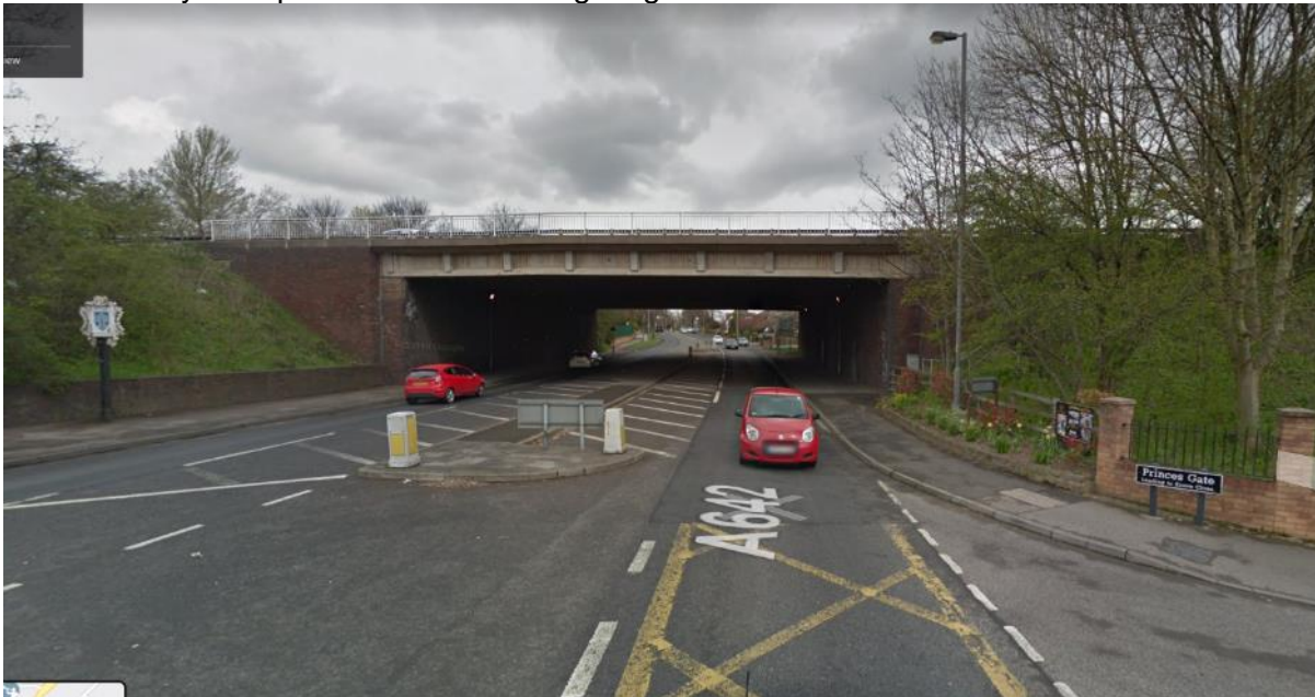
Figure 5.8 Horbury Road Bridge viewed from the west (source: Google Streetview, August 2020)
