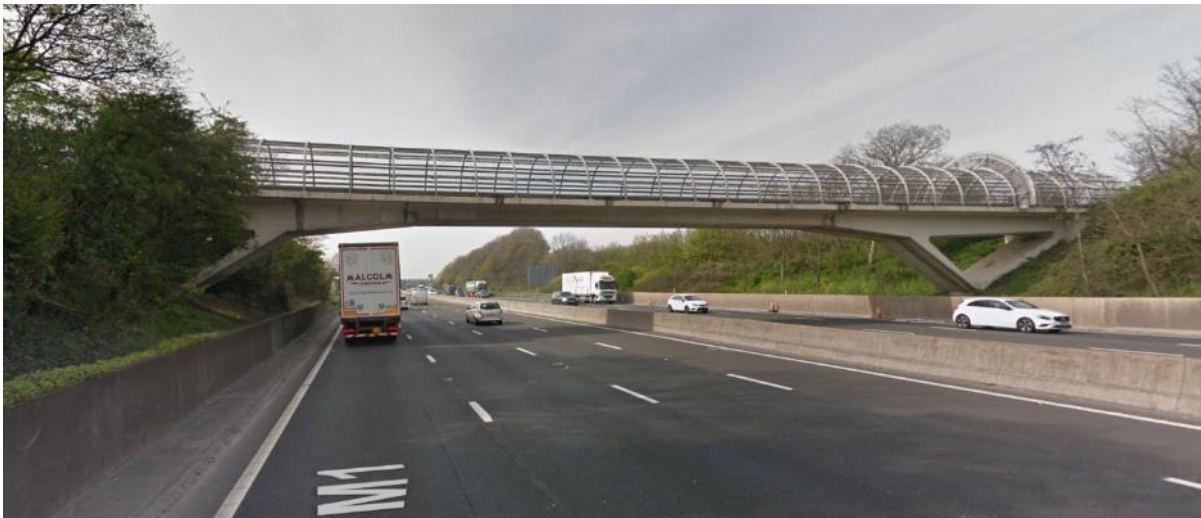
Figure 5.10 Snapethorpe Accommodation Bridge viewed from the south (source: Google Streetview, August 2020)
