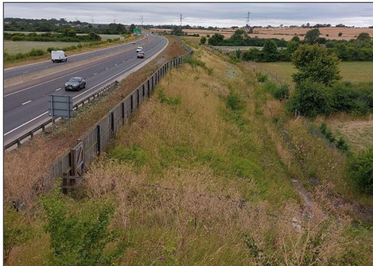
Figure 21 Noise barrier west of Grove Farm overbridge
