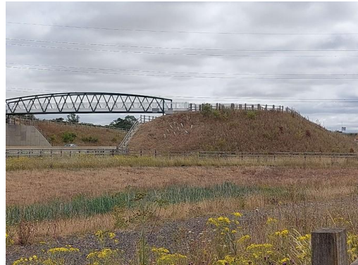
Planting not well established near footbridge 5
