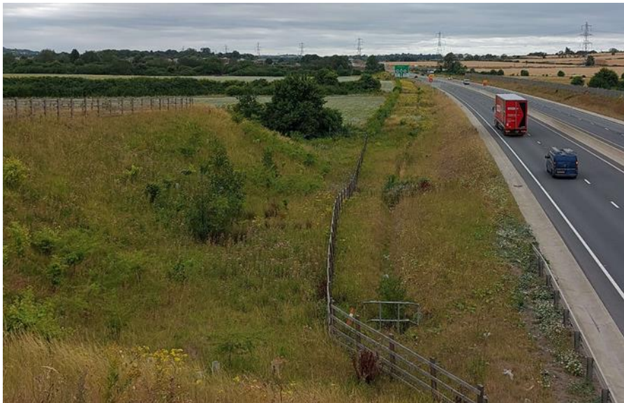
Figure 23 Landscape bund west of Grove Farm overbridge
