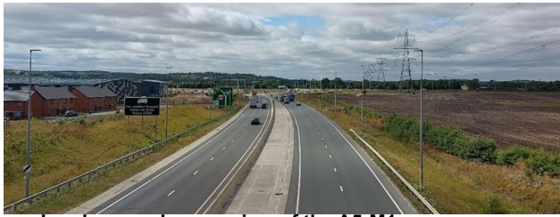
Landscape change: view of the A5-M1 southwest of Thorn farm overbridge
