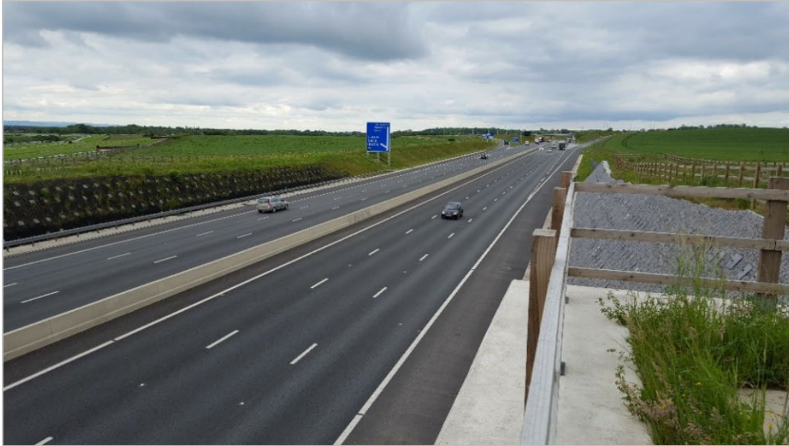
Figure 20 Fort Bridge Catterick Road July 2019 – south side
