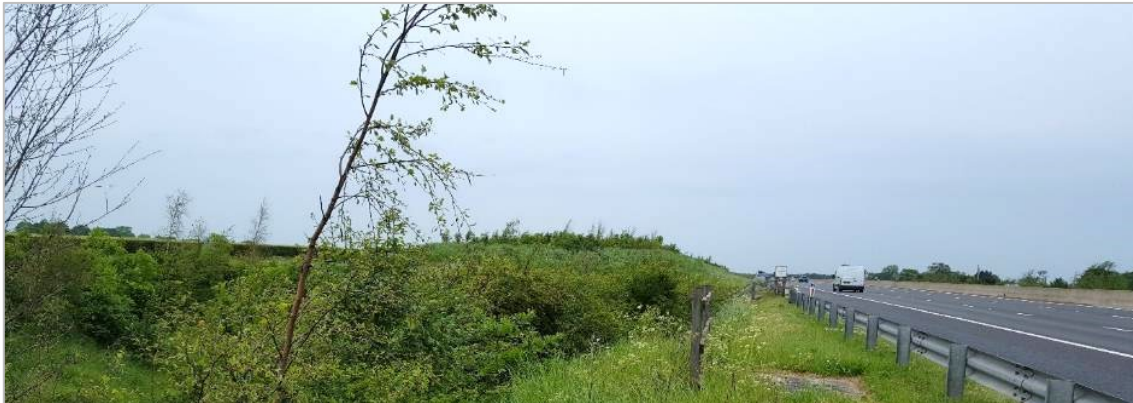
Figure 17 Landscape bund at Oak Tree underpass 7YA
