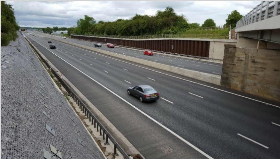
Figure 19 Fort Bridge Catterick Road July 2019 – north side
