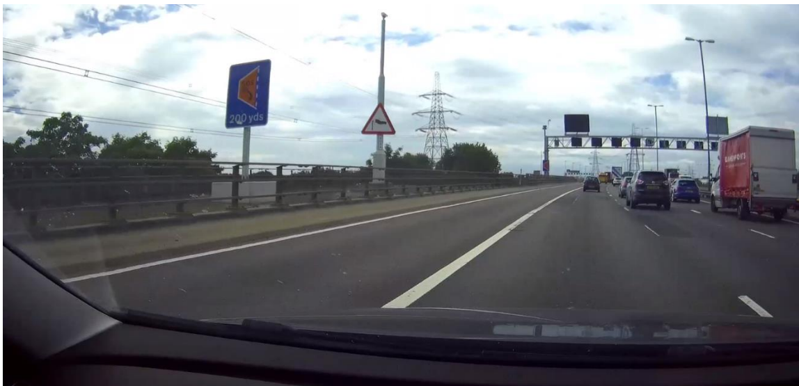
Figure 5.2 View of northbound emergency area at 200 yards sign.
