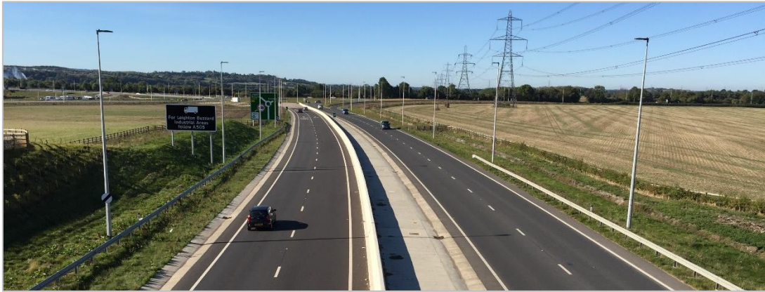
Fig 14 Lighting columns near the A5 roundabout
