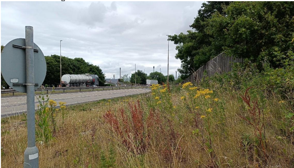
Figure 25: Noise barriers on either side of the A160
