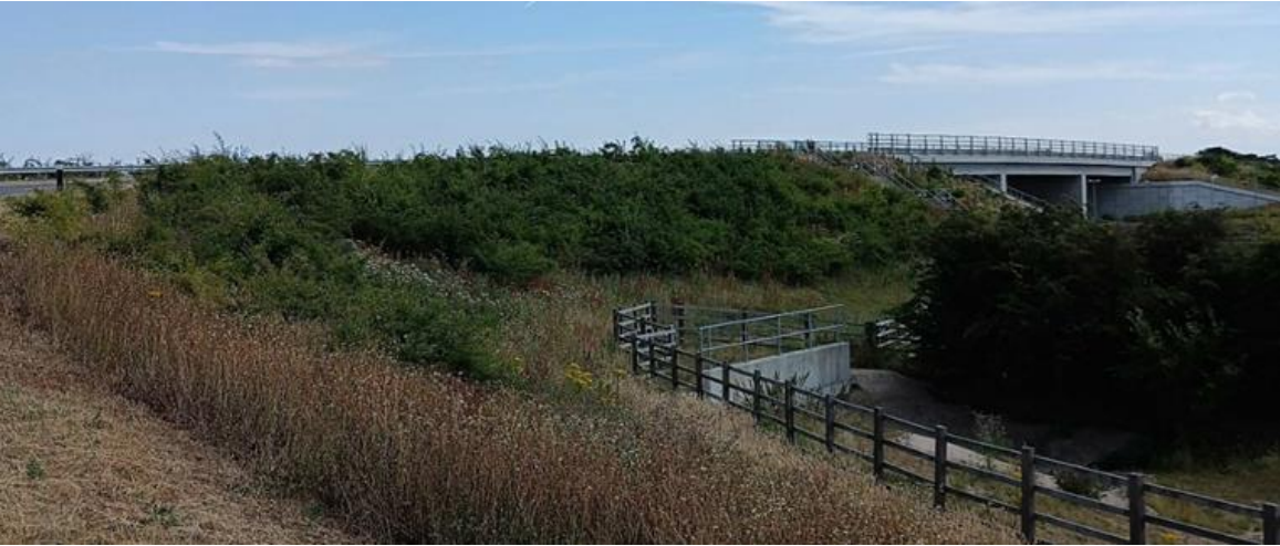
Source: Five-year after evaluation site visit (July 2022).
