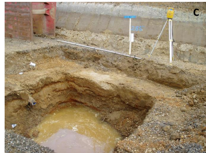
Figure 16. Belhus Park cutting: A: Clayey/silty organic-rich channel-fill above Corbets Tey Gravel, dipping north. B: Belhus Cutting organic-rich channel-fill below fluvial sand/gravel deposits. C: fluvial sand/gravel beds in bottom part of Belhus Cutting organic-rich channel.
