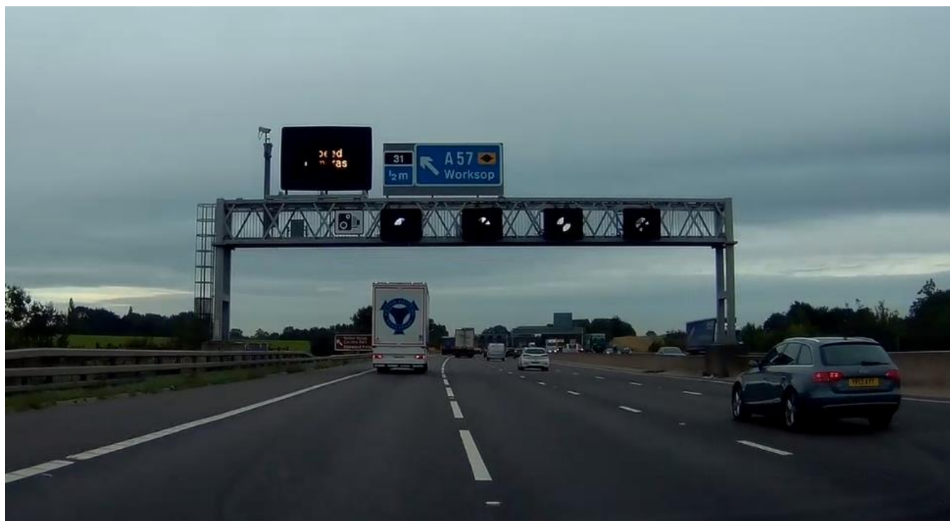
Figure 5.6 ½ mile advanced direction sign for Junction 31 over lane 1 / 2; hazard lines between lane 1 / 2 (dashcam video, July 2020)
