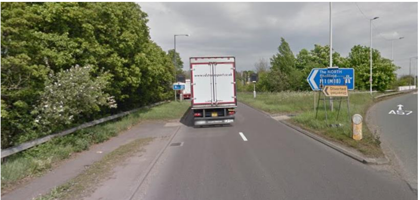
Figure 5.11 Streetview image of Junction 31 northbound entry slip
