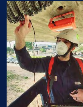
Example of testing on anchorage wires
