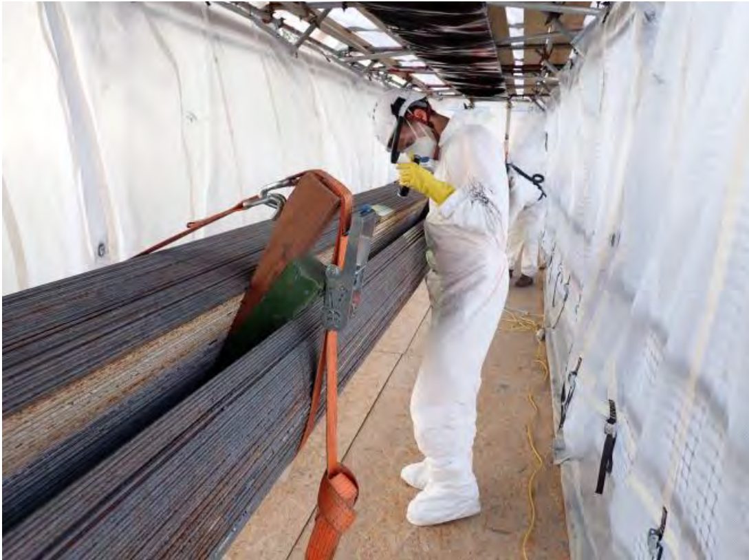
Suspension Bridge Cables
