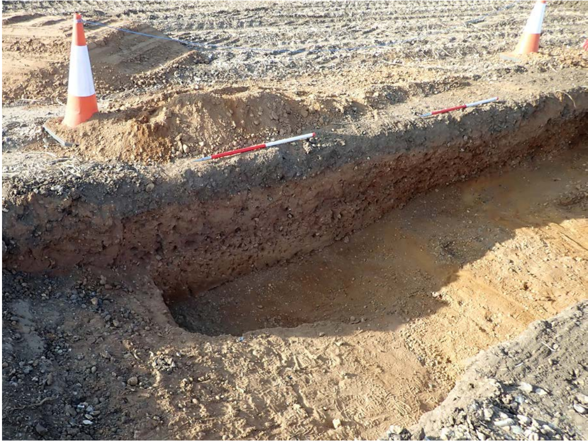
Plate 8: Section 12802, looking south west
