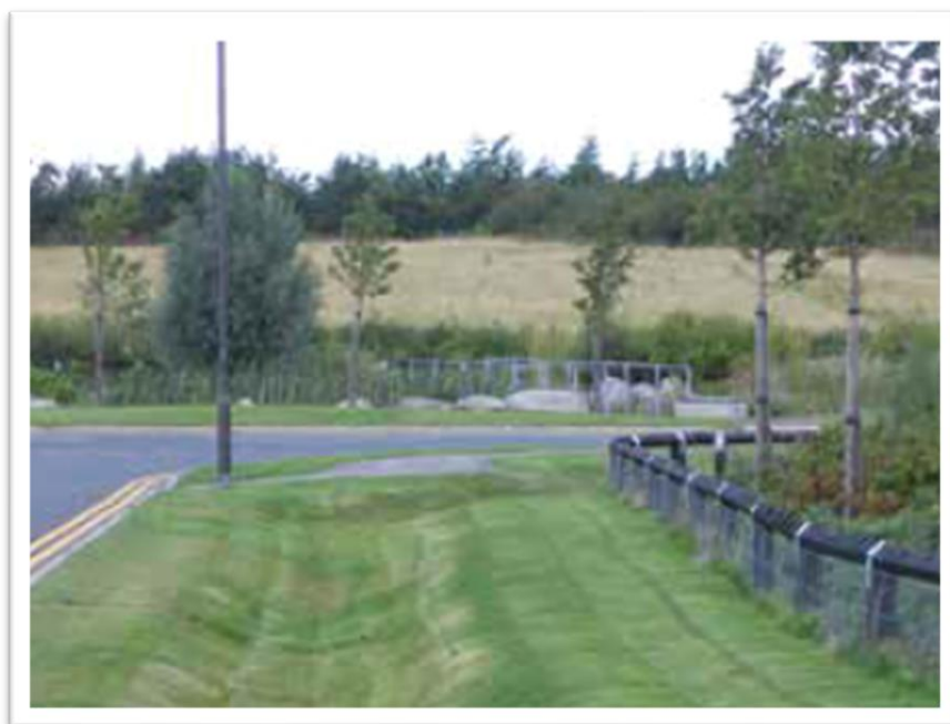
Figure 3-4 – Typical swale
