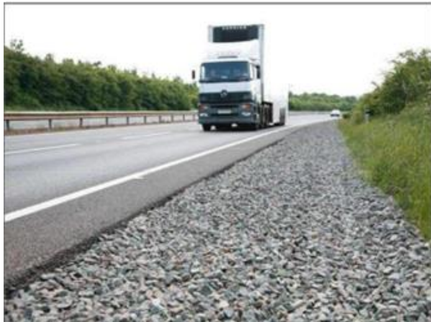
Figure 3-5 – Typical filter drain
