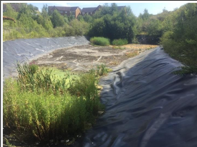
Large balancing pond with an exposed liner with inflow from the adjacent housing estate. Largely dry but with two areas of shallow standing water one at each end supporting bulrush, club rush, great willowherb, and purple loosestrife. Surrounding area is completely unmanaged with patches of calcareous ephemeral/short perennial habitat rapidly succeeding to scrub and woodland. Cotoneaster and buddleia are particularly widespread.
