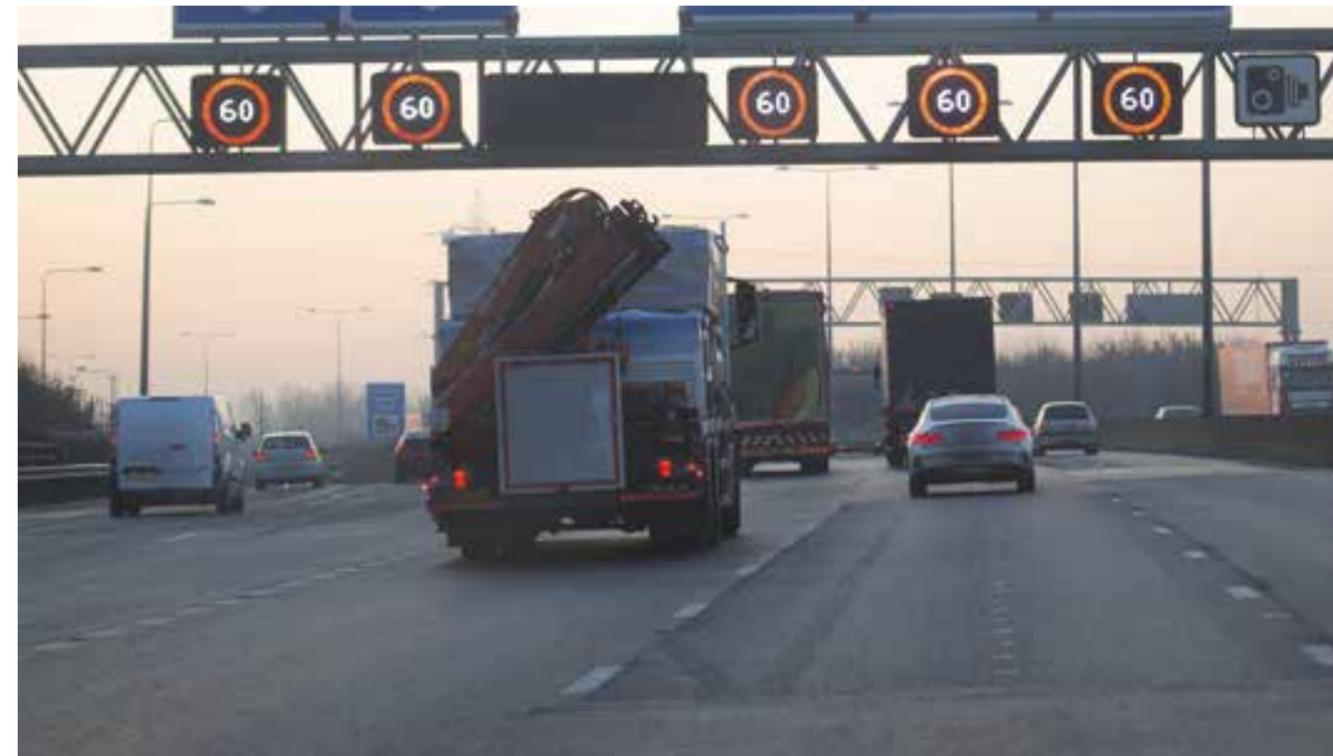
Figure 7 Variable speed limits in operation
