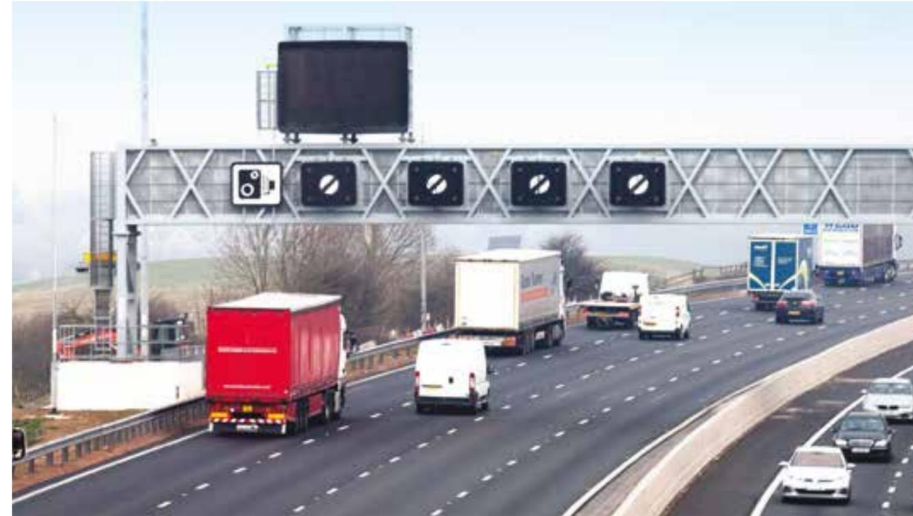
Figure 8 National speed limit displayed on signals
