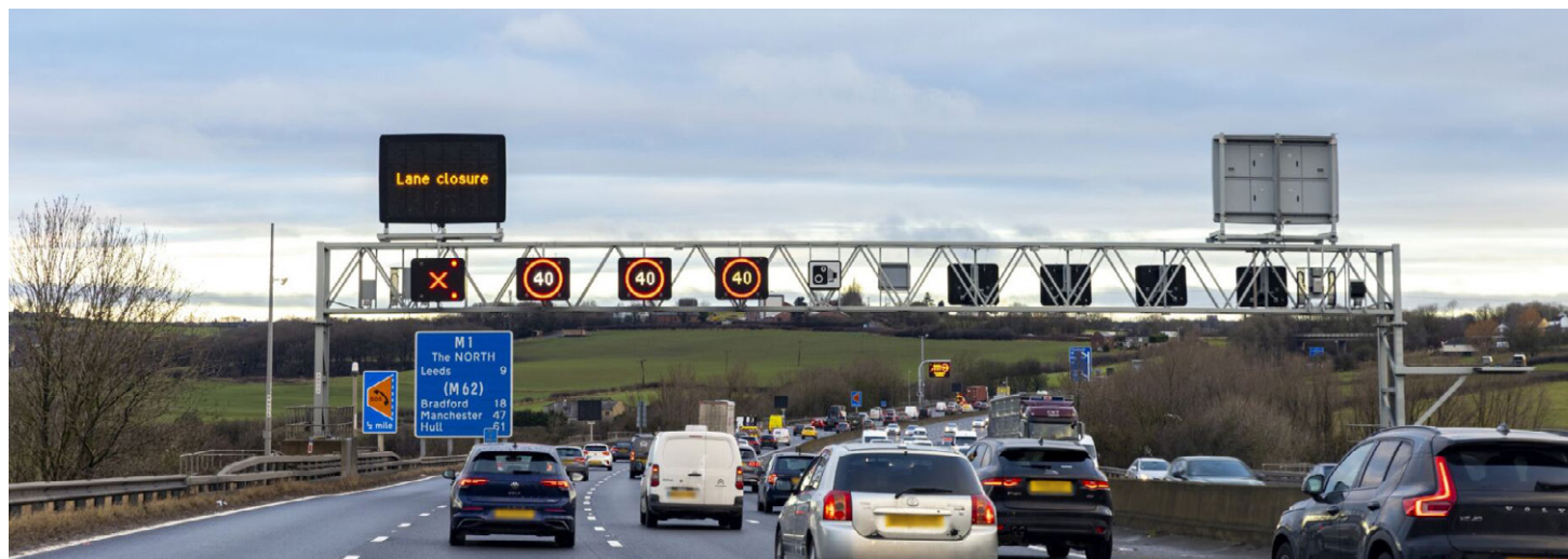
Red X and lane closure sign in use on ALR motorway
