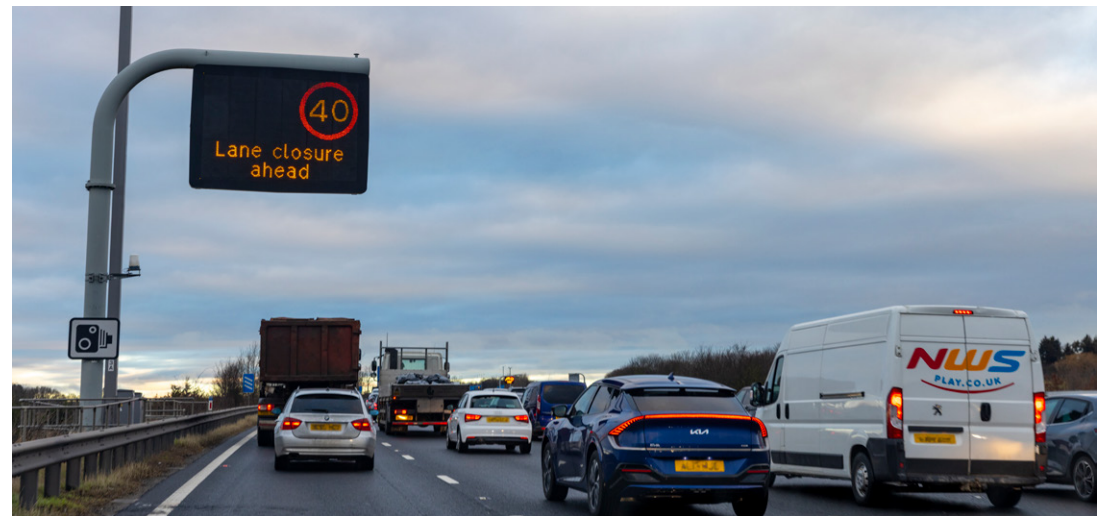
Sign and signal in operation on ALR motorway
