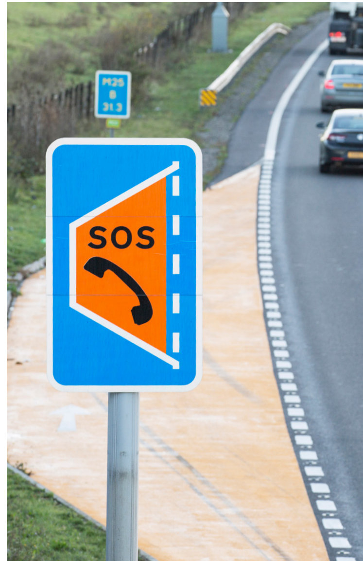
Emergency area and sign
