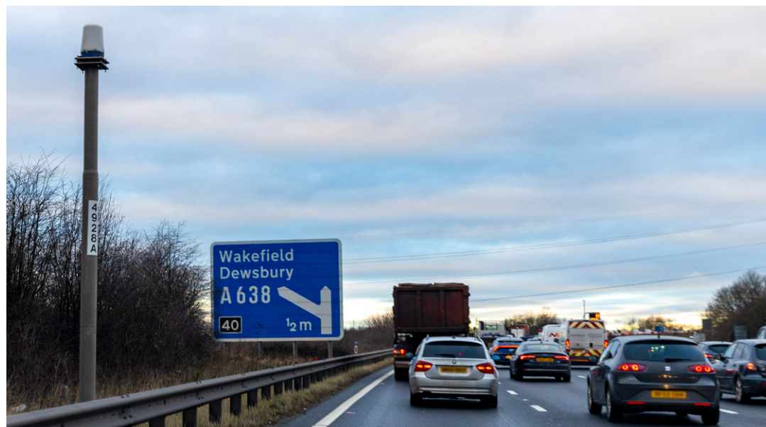
SVD technology on ALR motorway
