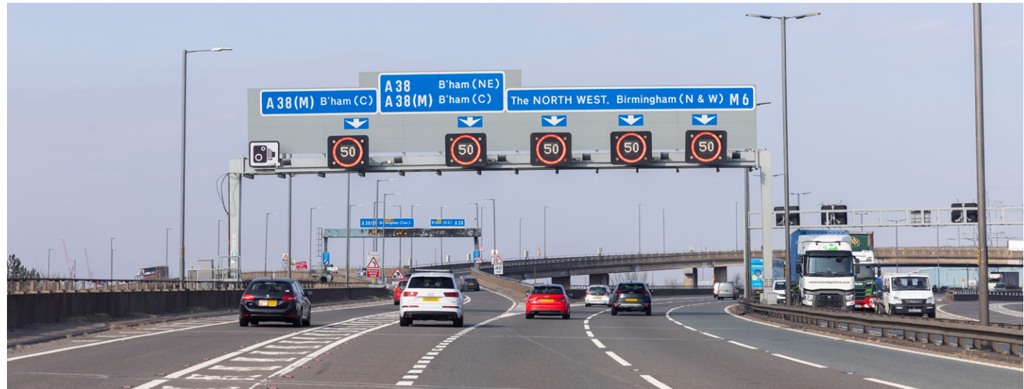
West Midlands DHS motorway junction
