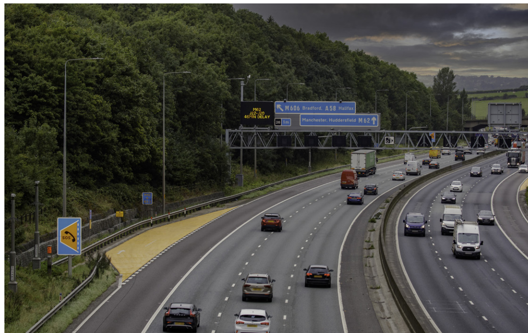
DHS motorway in West Yorkshire
