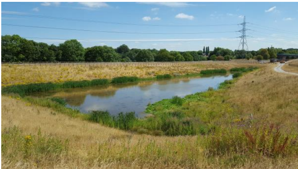
Figure 12 Balancing pond near the Bowdon junction
