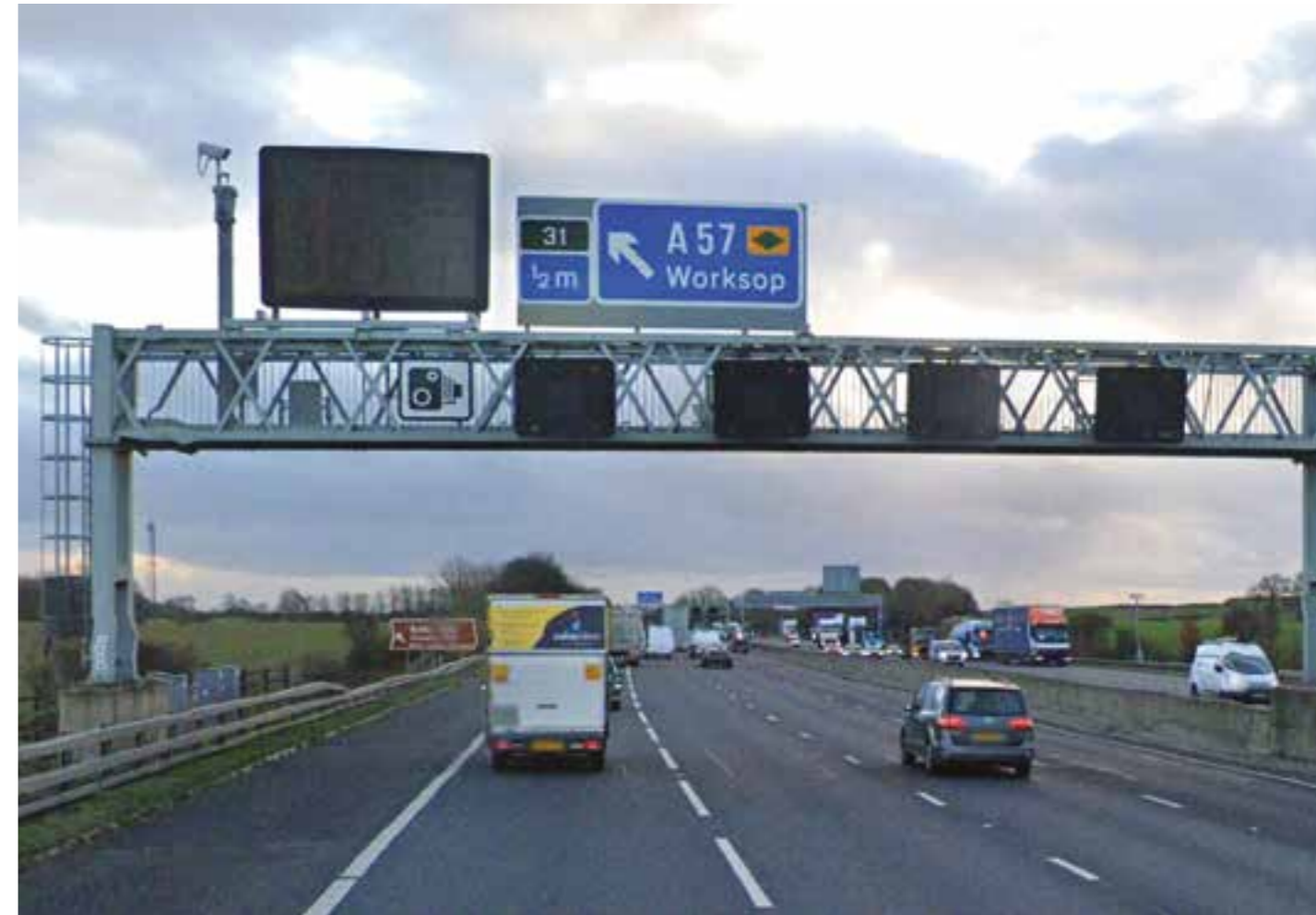
Figure 2 M1 J31 southbound ½ mile advance direction sign and hazard road markings between lane 1 and 2 © Google
