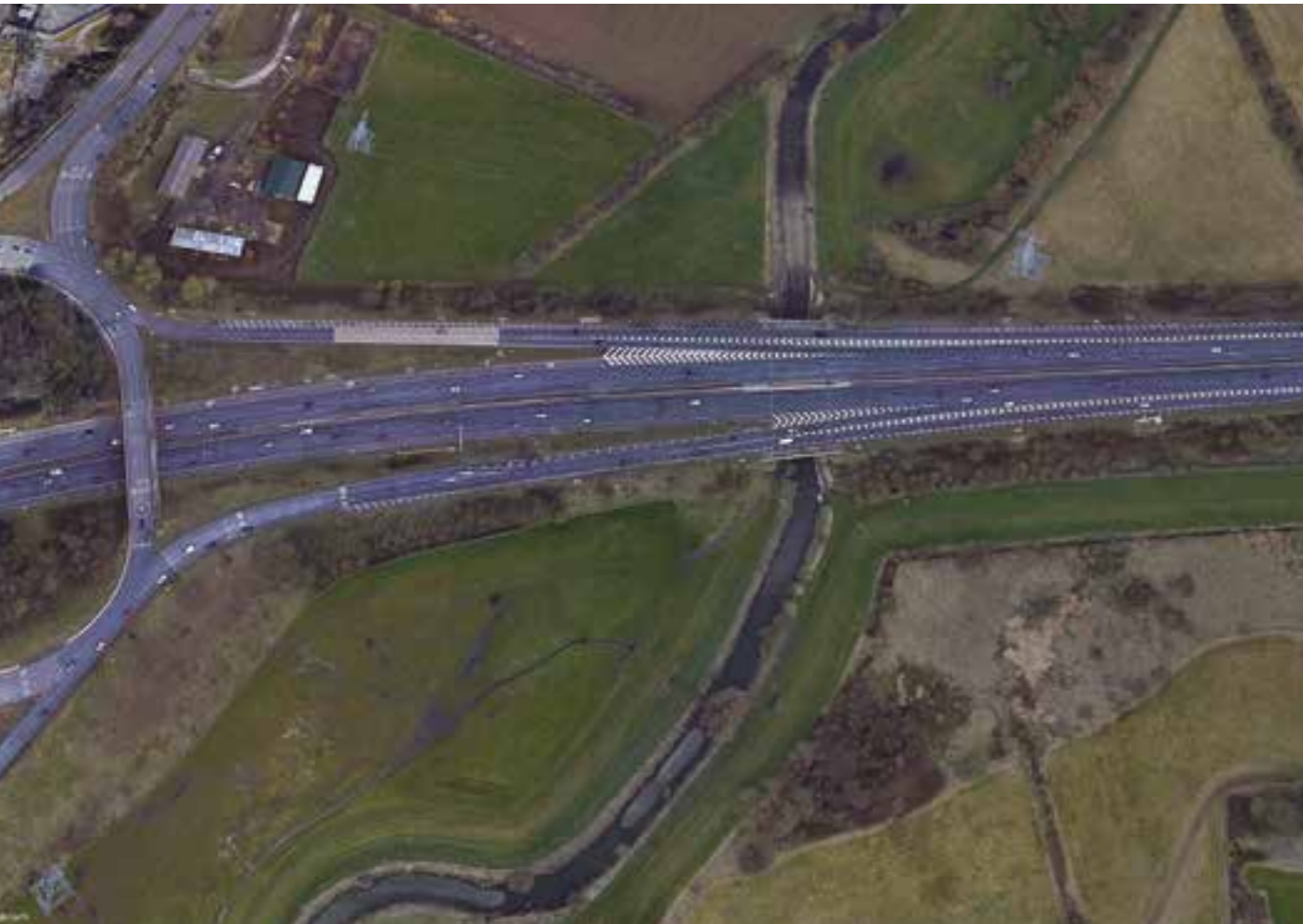
Figure 1 M1 J33 northbound exit slip road (shown on lower portion of image) © Google
