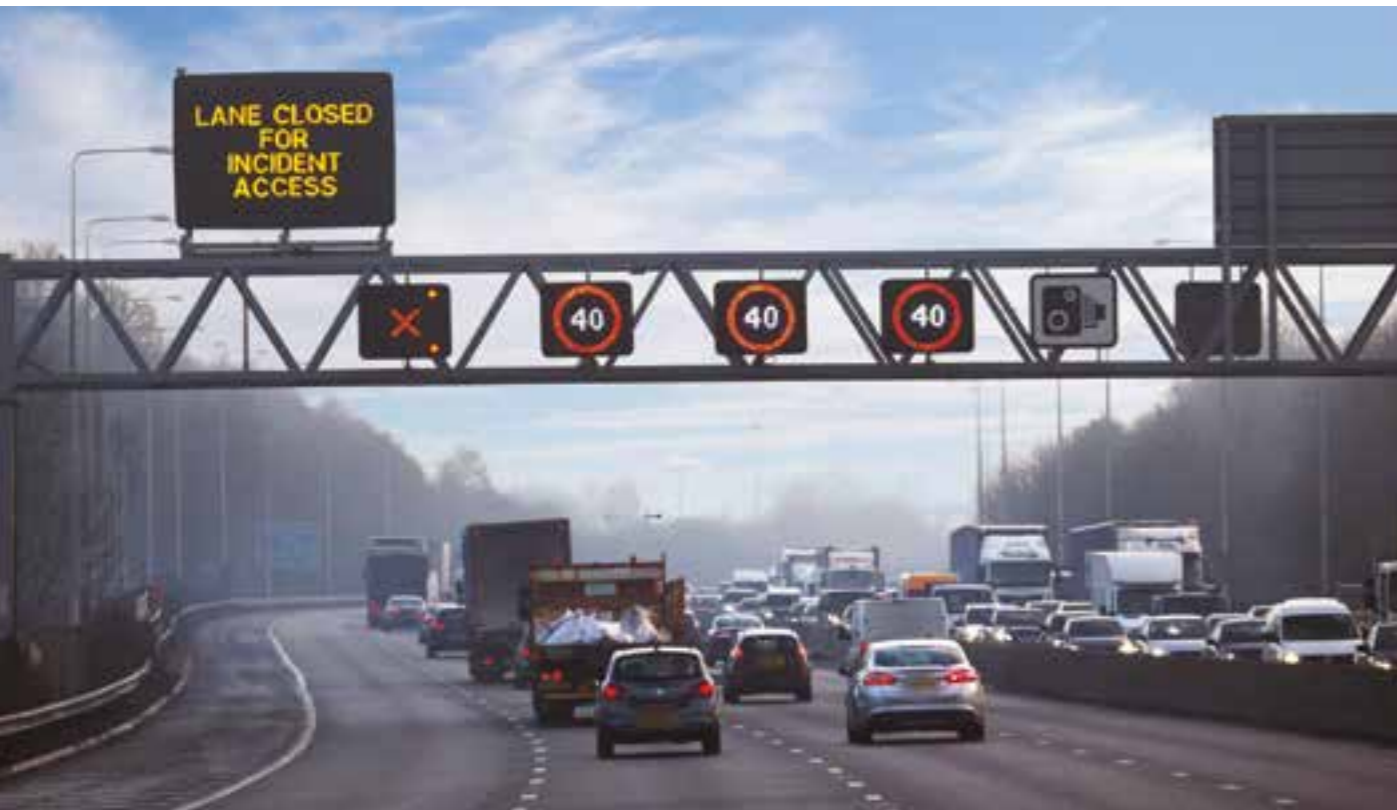
Figure 5 Signs and signals used on a section of smart motorway
