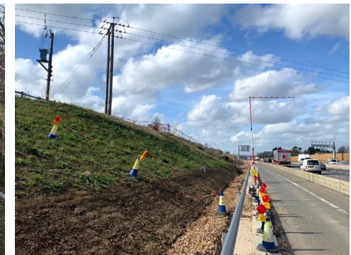
Blue cones for overhead services hazard warning.
