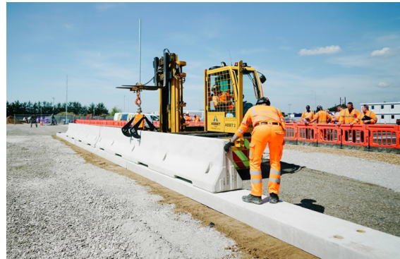
Precast barrier installation, drilling and pinning trial in DHS M40/M42 compound, May 2022.
