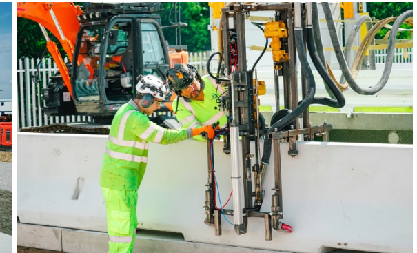
Precast barrier installation, drilling and pinning trial in DHS M40/M42 compound, May 2022.
