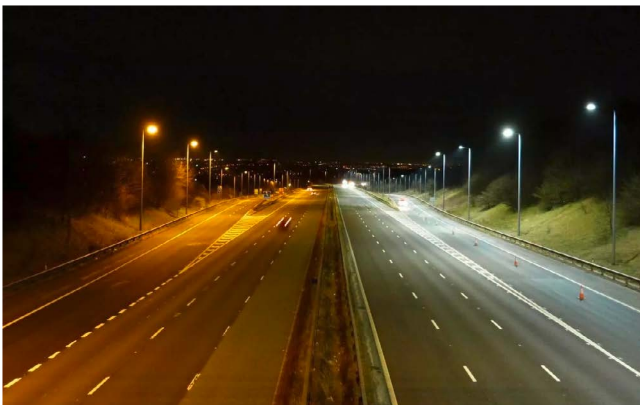
Figure 10: LED lighting (white) vs. traditional sodium lighting (orange) on the M62 in Yorkshire
