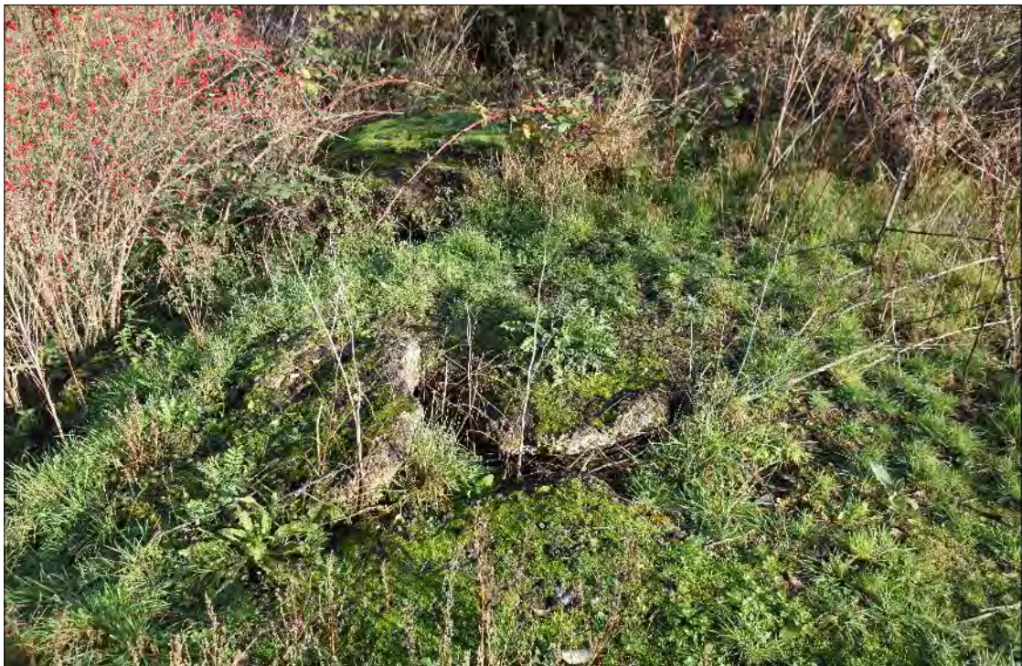
Plate 18: Orsett: concrete identified in the eastern section of the eastern field, facing west
