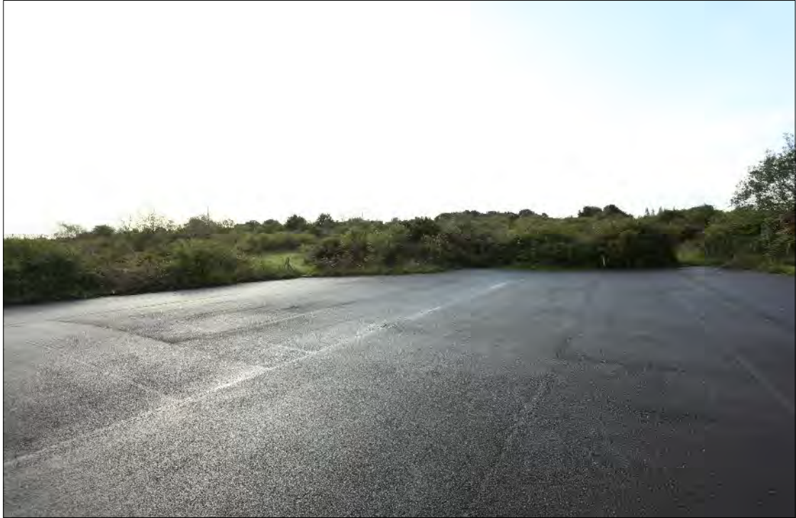
Plate 5: Orsett: view of Whitmore car park, facing southwest
