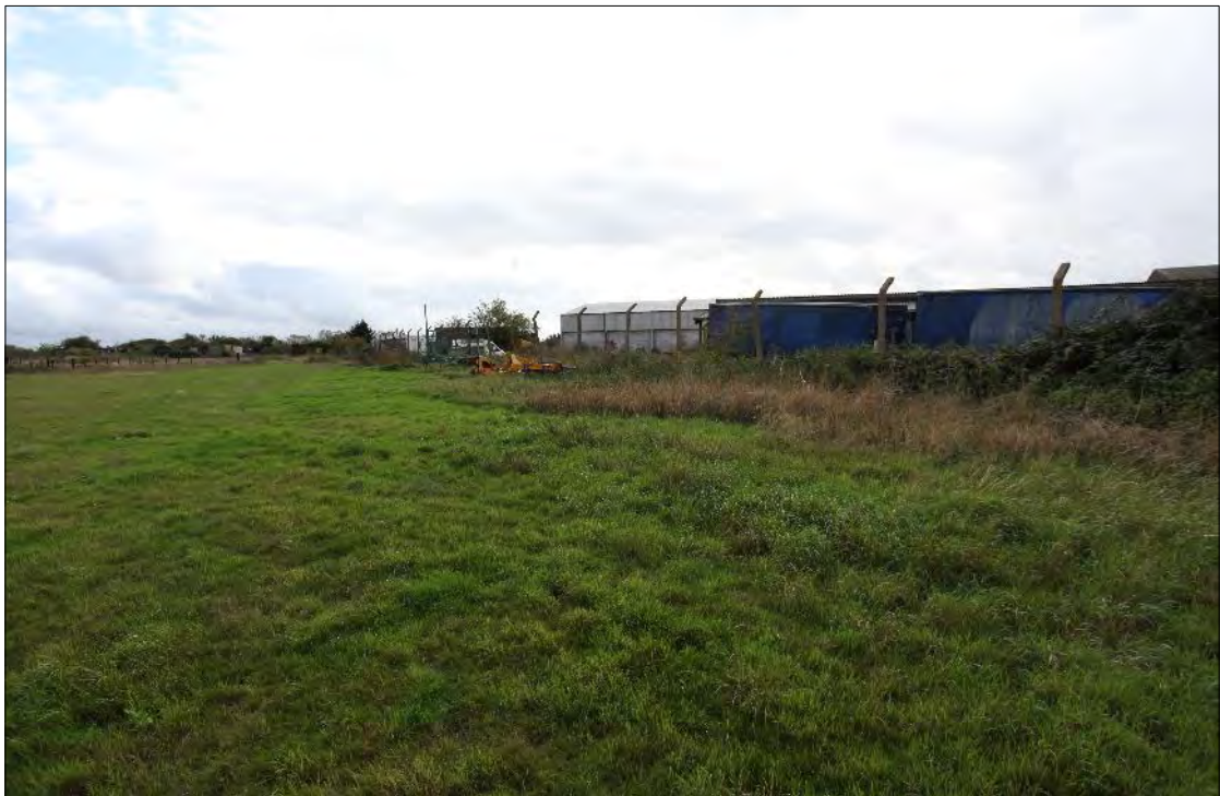
Plate 46: Bowaters Farm: view of surviving concrete boundary fence posts along the Western boundary, facing southwest
