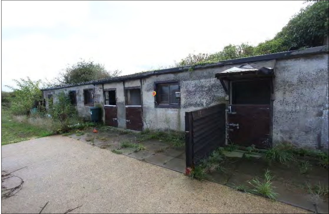
Plate 35: Bowaters Farm: view of former storage buildings, facing southeast
