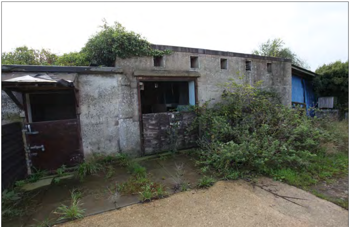
Plate 34: Bowaters Farm: View of former generator building, facing southwest
