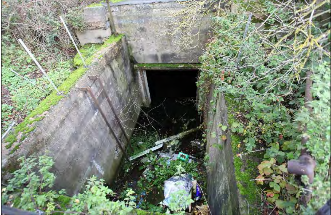
Plate 41: Bowaters Farm: View of 5.25inch gun emplacement entrance with its surviving iron ladder, facing southeast
