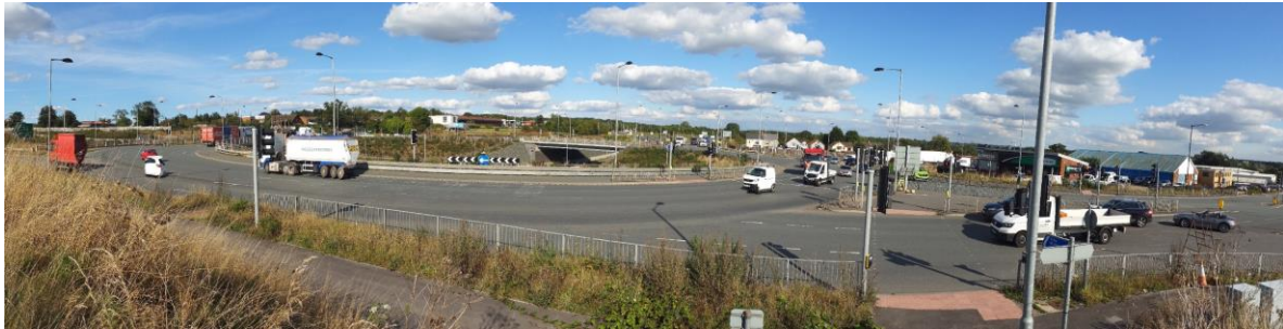
Figure 31 The grade separated Tollbar End junction at five years after
