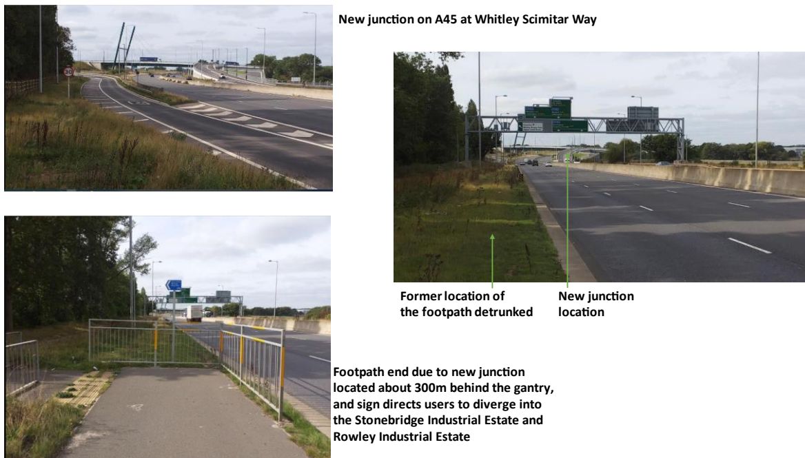
Figure 30 Landscape changes along Stonebridge highway after the project
