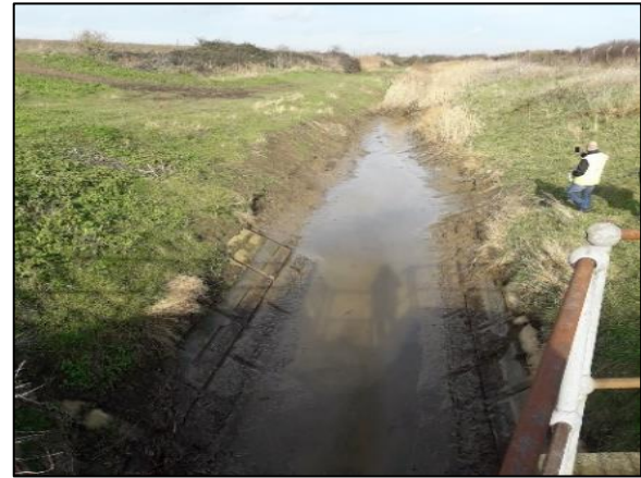
View 4: North view from the top of Bowaters Sluice showing West Tilbury Main.
