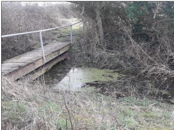
View 3: Orsett Fen Sewer (ref. F)
