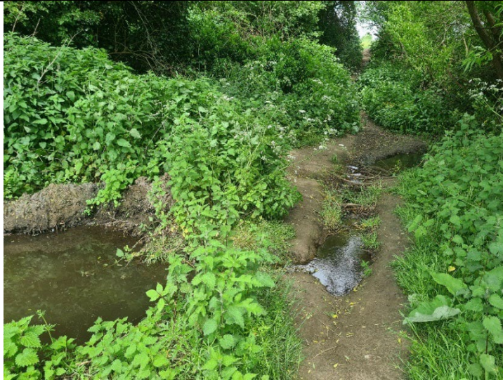
High water level was noted in the drainage ditch along the northern border of both fields (photo taken at intersection of the western and eastern field)
