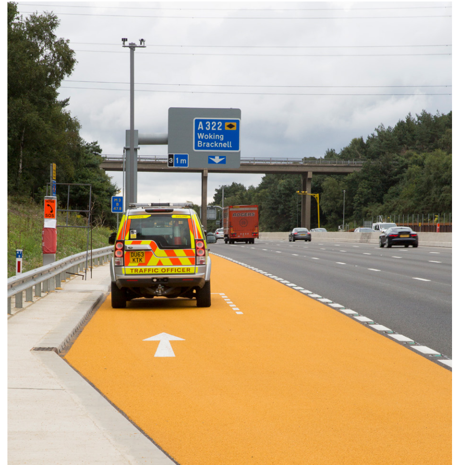
National Highways traffic officer vehicle in an emergency area
