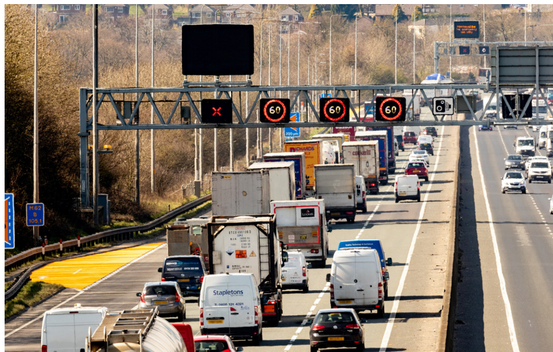
M62 junction 27 dynamic hard shoulder motorway
