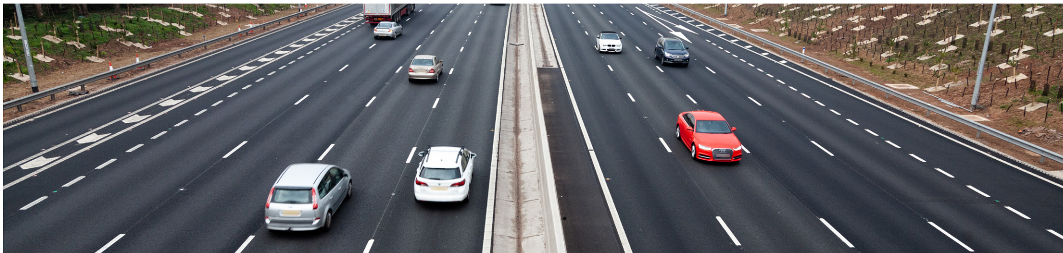
All lane running motorway on the M1
