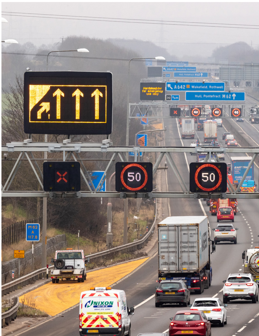
M62 junction 30 dynamic hard shoulder motorway
