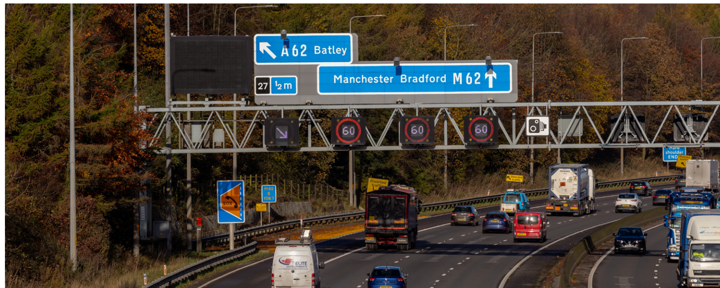
M62 junction 27 dynamic hard shoulder motorway
