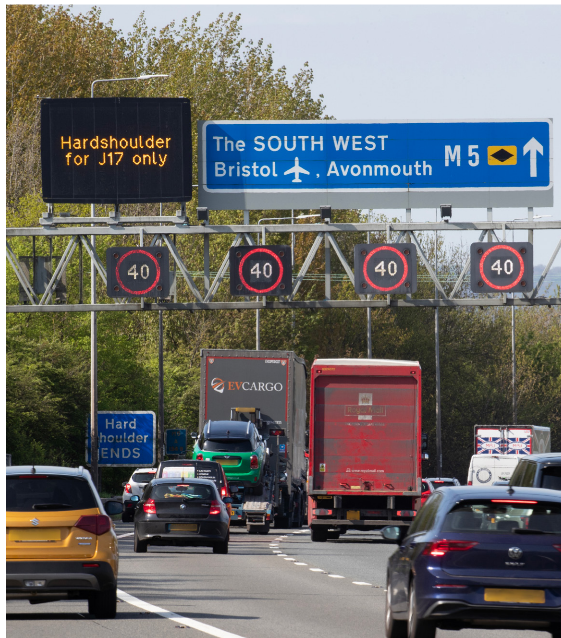
M5 junctions 16 to 17 dynamic hard shoulder motorway
