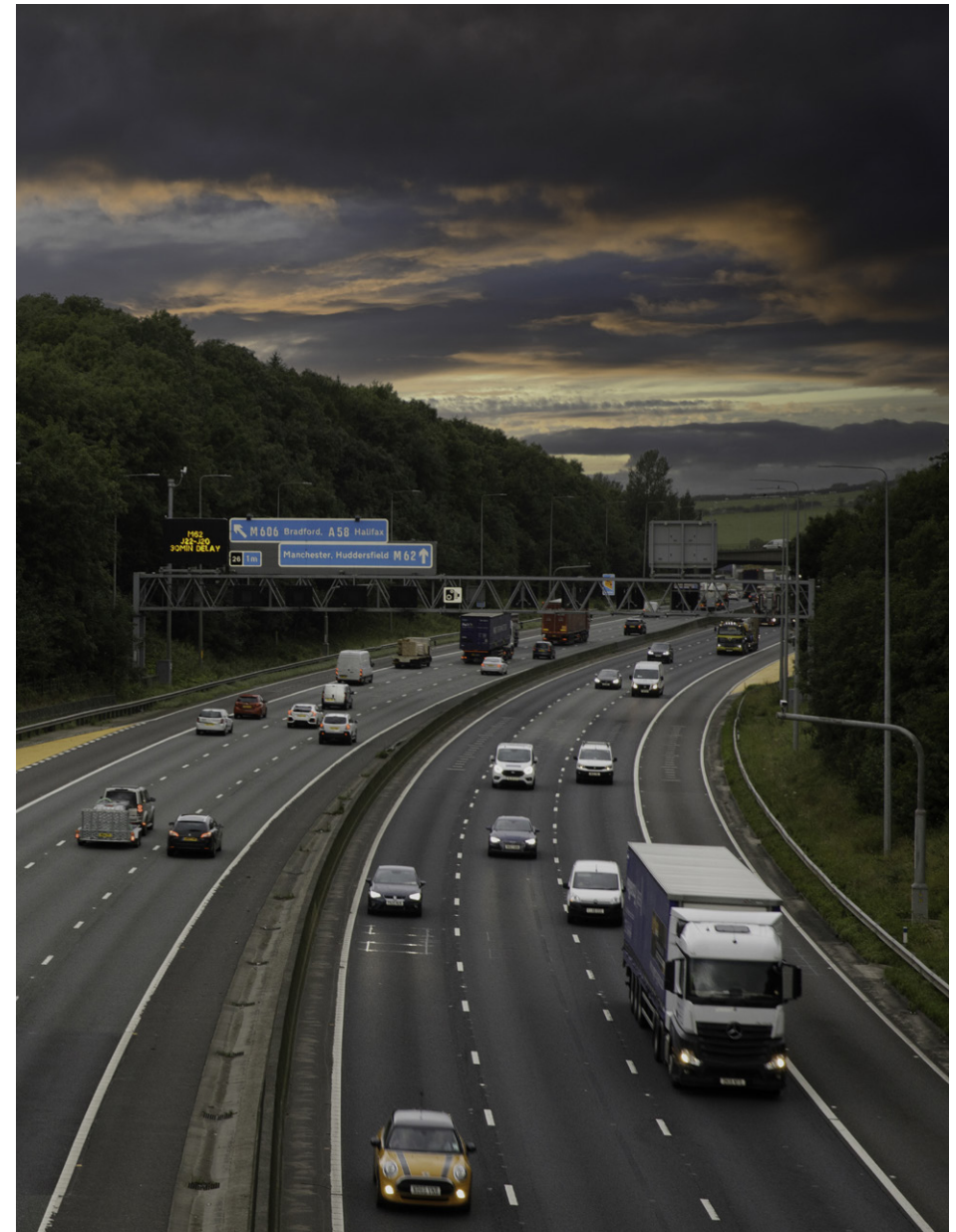
M62 junction 26 dynamic hard shoulder motorway
