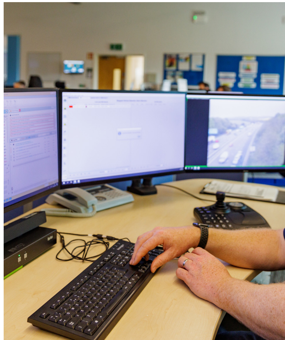
An operator's desk in a National Highways' control room
