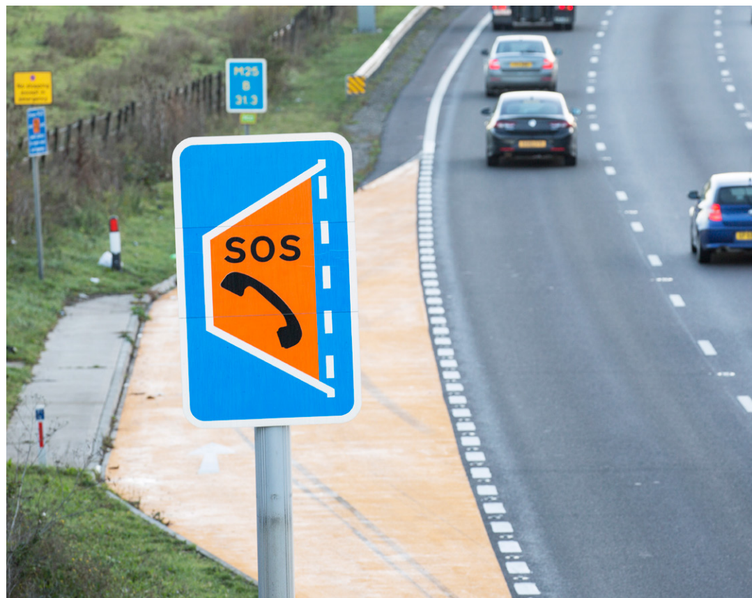
Emergency area and sign
