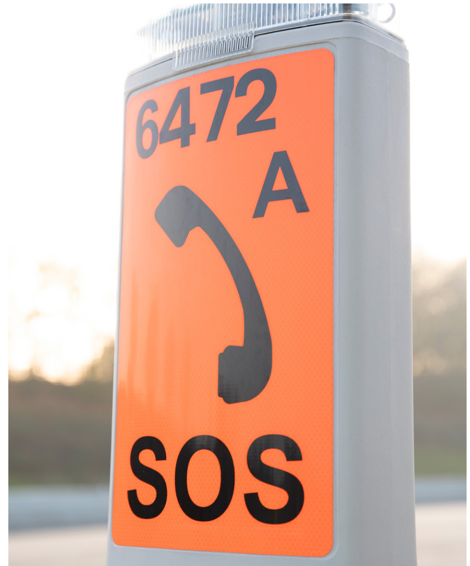
Emergency roadside telephone
