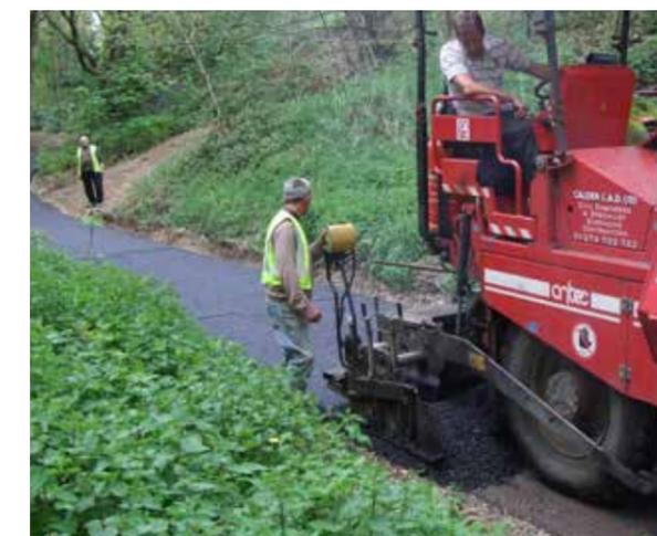
Figure 70. Greenway construction site, Sustrans
