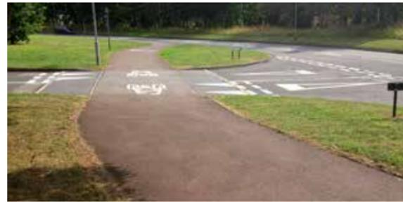
Figure 52. Illustration of a bent-out crossing. Source <https://www.cycling-embassy.org.uk/wiki/a-question-of-priority>
