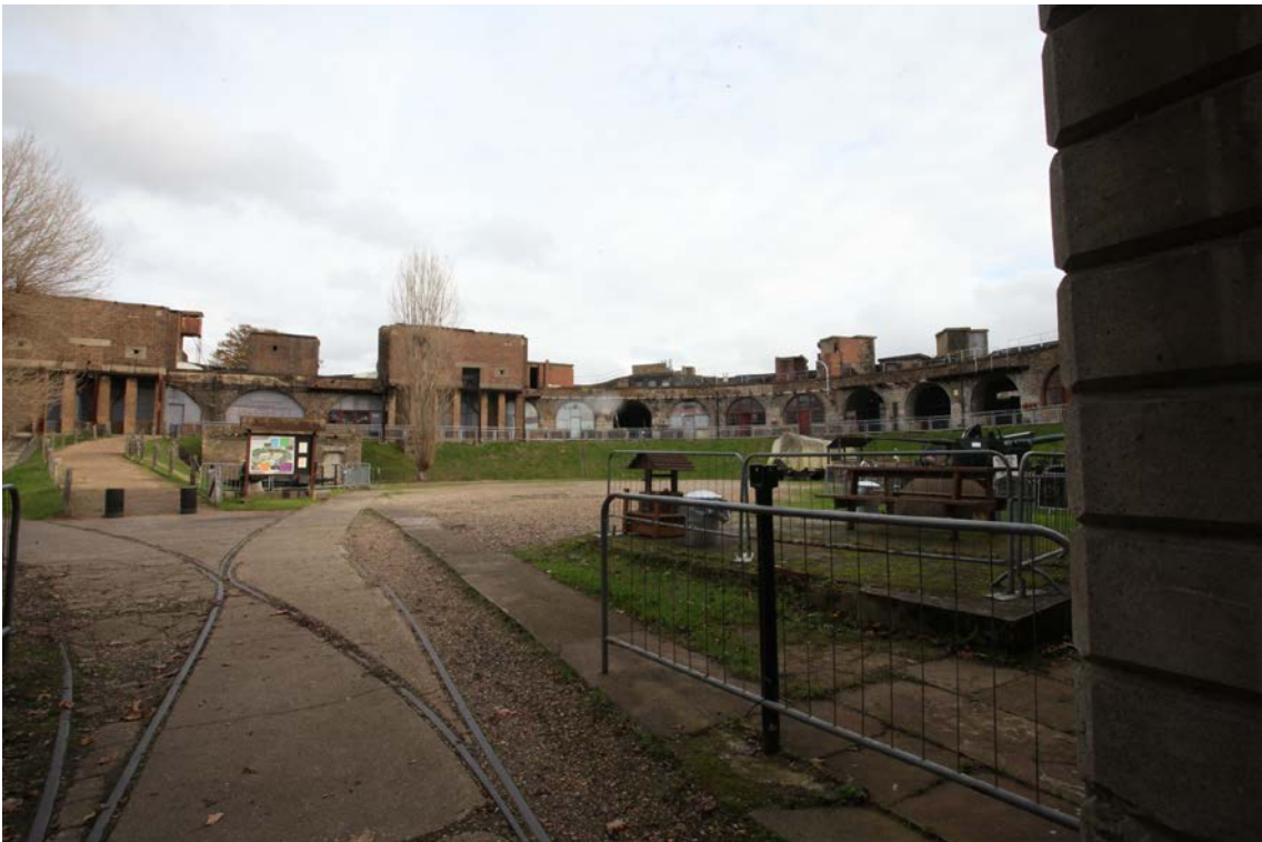
Plate CHF2: Interior of Coalhouse Fort
