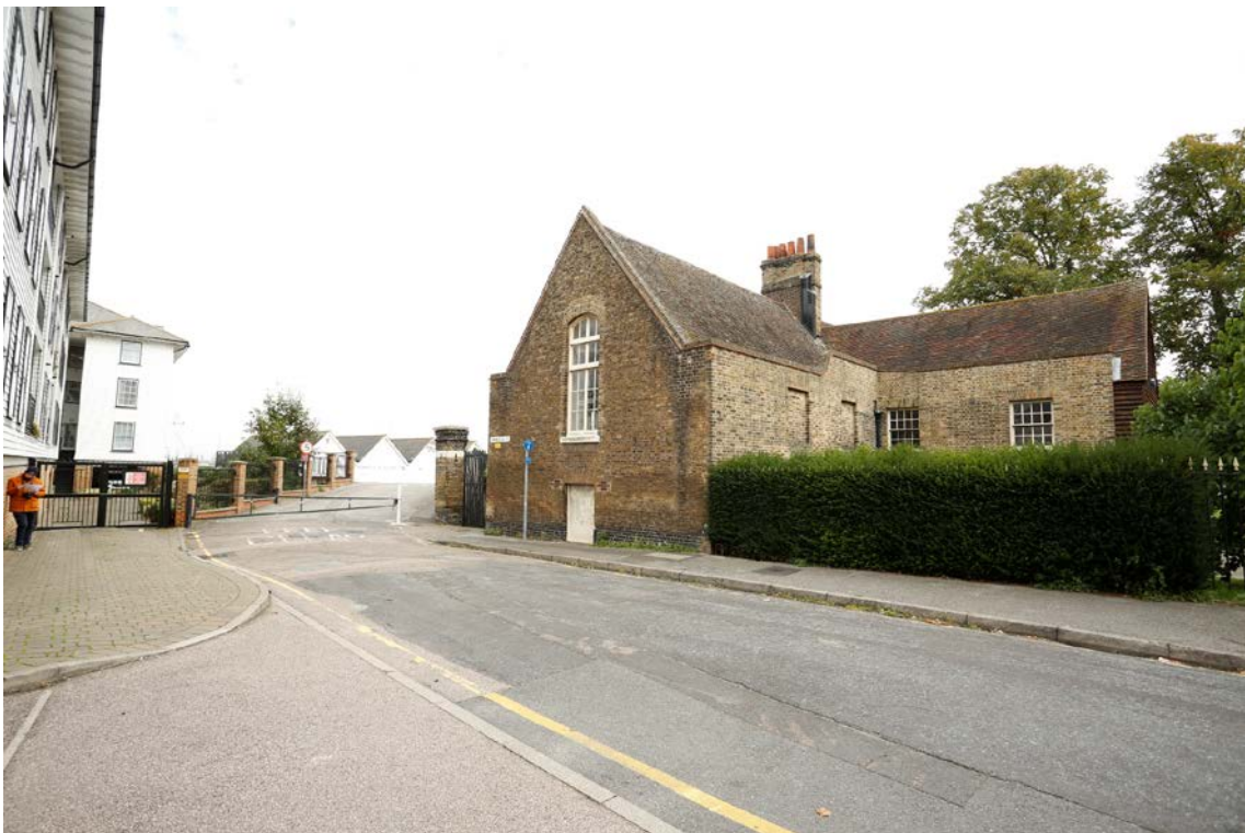
Plate NTF2: Milton Chantry viewed from the south-west
