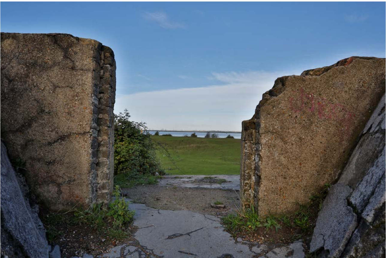
Plate SF6: View from the open battery towards Tilbury Docks
