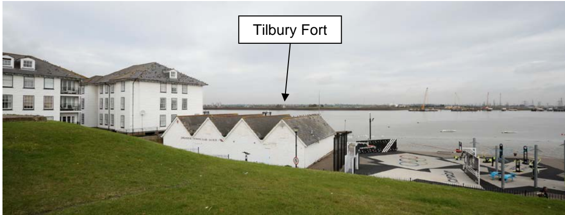
Plate NTF8: View from 6-inch gun emplacement on the angled battery looking towards Tilbury Fort
