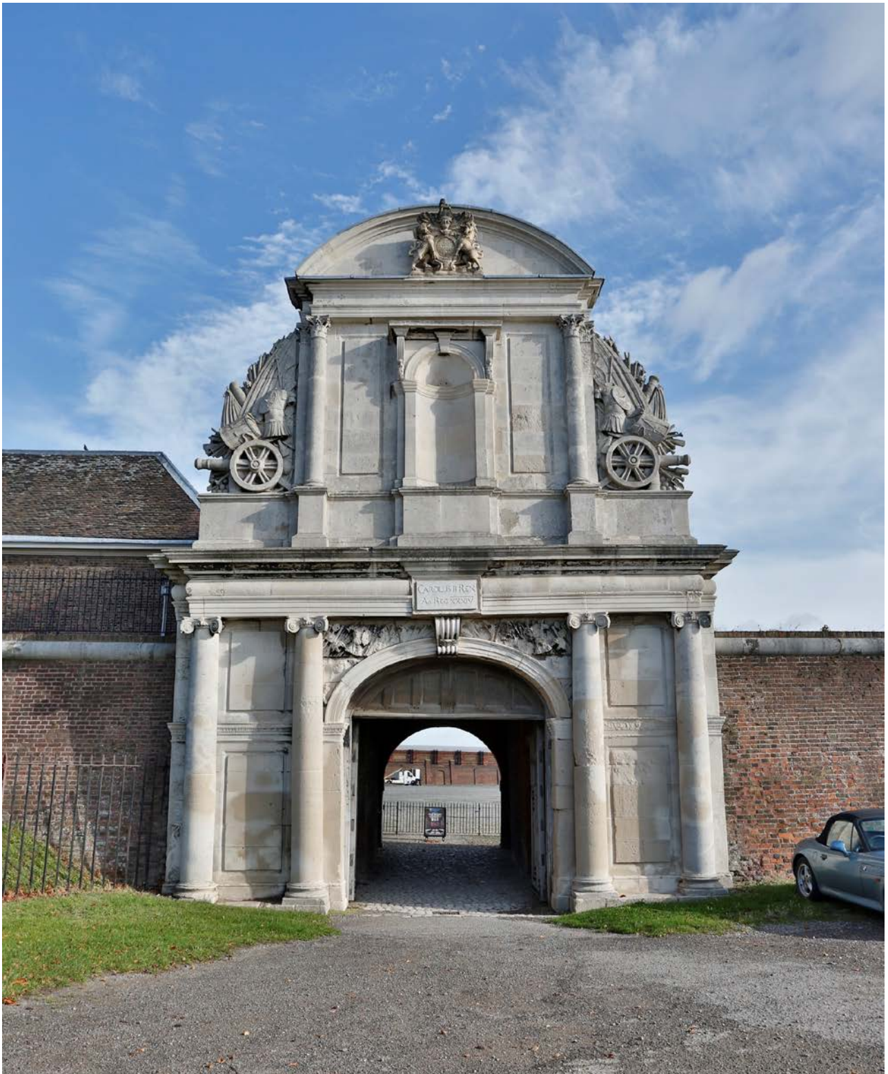
Plate TF1: Tilbury Fort Water Gate
