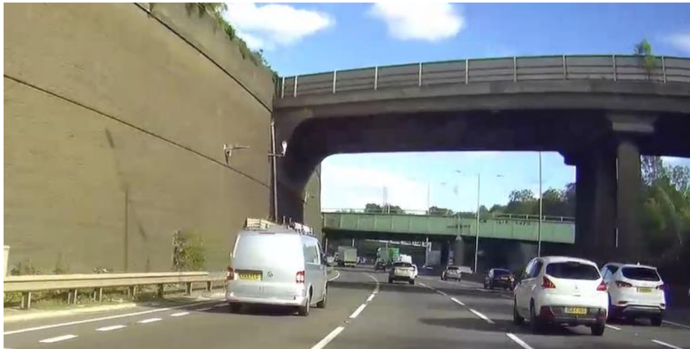
Figure 5.10 View southbound at junction 11 merge tip (Dashcam footage July 2020)
