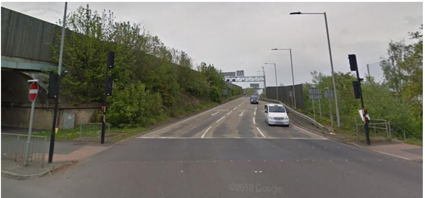
Figure 5.4 StreetView image of junction 11 southbound exit slip
