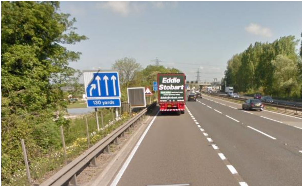
Figure 5.1 View of advance signing associated with the transition from through junction running to dynamic hardshoulder
