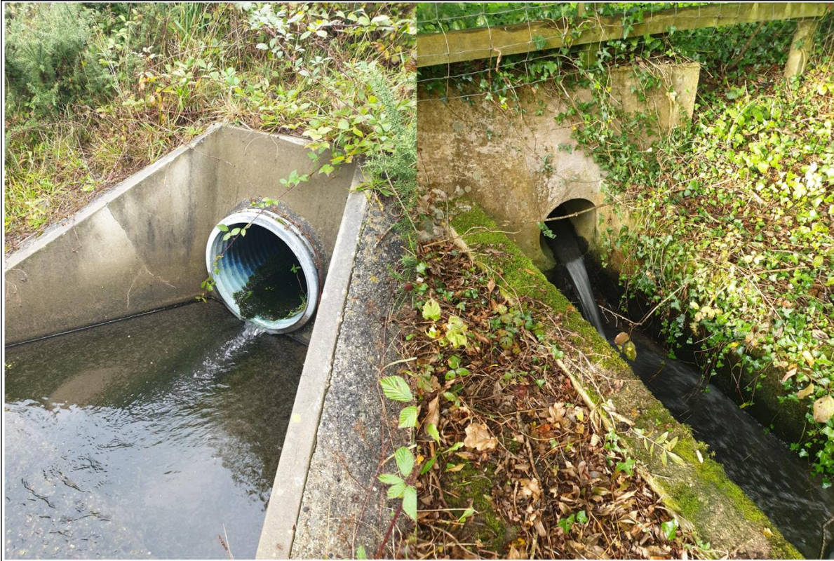
Figure A.3: Example of drainage points at which water samples were collected from a retention pond inlet (left) and a direct drainage outfall (right). Source: Florence Parker-Jurd University of Plymouth, 2022.
