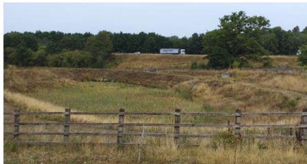
Balancing pond one at 5YA (Source: 5YA Evaluation visit August, 2022)
