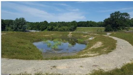
Balancing pond one at 1YA (Source: 1YA Evaluation Report, February 2020)
