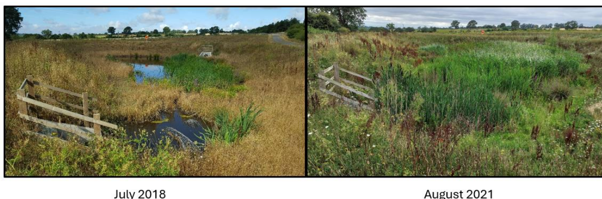
Figure 26 Example of heavily vegetated drainage network (including by the drainage inlet)
