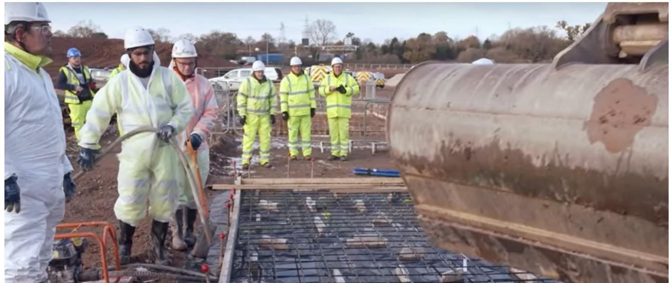
*Trialling low carbon reinforced concrete on a temporary access road at junction 6 of the M42*
